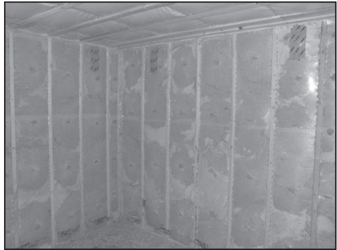
Figure 3. Double walls after cellulose insulation. Image courtesy Steven Winter Associates.
