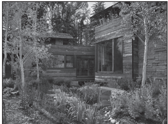
Figure 10. In unison with the native landscape, exterior home elements include reclaimed snow fence and locally quarried stone. Image courtesy Roger Wade.
