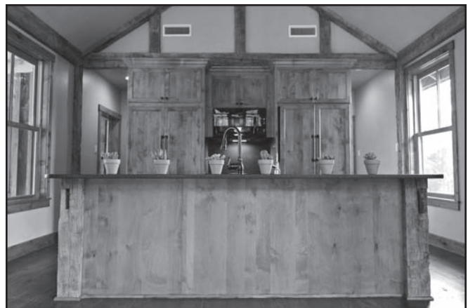
Figure 6. Cabinets at the Casita are certified formaldehyde-free, and flooring and interior wood beams are sourced from reclaimed lumber. Image courtesy Travis Laminack Photography.
