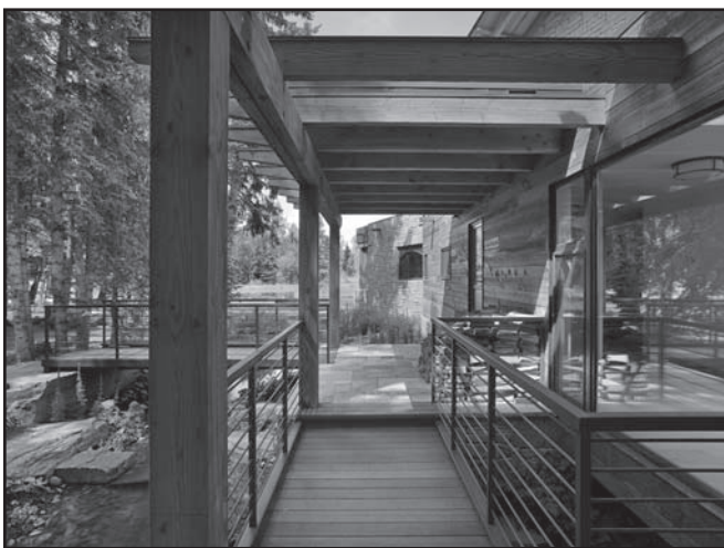
Figure 9. Dividing the home into smaller buildings meant more comfortable, easier to heat spaces. Bridges between the home’s elements contribute to aesthetics and offer integrated overhangs. Image courtesy Roger Wade.
