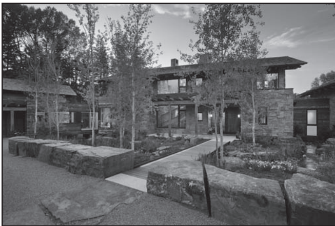
Figure 8. The John Dodge Compound groups around a southern courtyard to maximize warmth and natural light. Native landscaping incorporates into the shading and seasonal solar heat gain scheme. Image courtesy Roger Wade.
