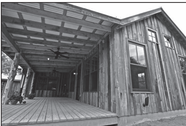
Figure 5. The porch and window positioning allow for strategic passive solar gain in the winter, while minimizing direct heat gain in the summer. Image courtesy Travis Laminack Photography.
