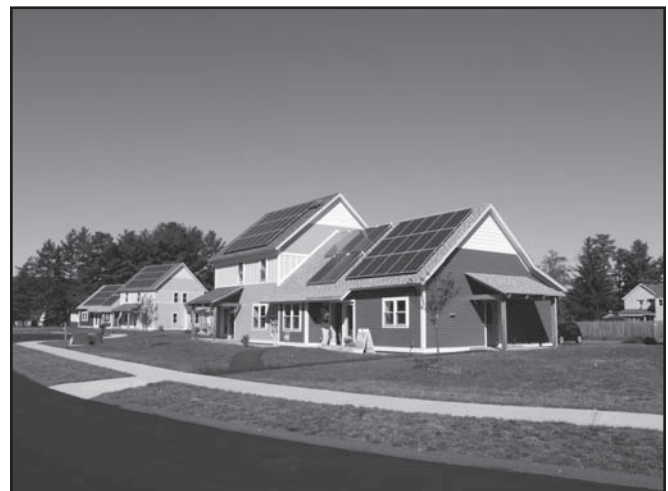
Figure 1. Rural Development, Inc. desired a whole community of near-zero homes for Wisdom Way Solar Village. Image courtesy Steven Winter Associates.
