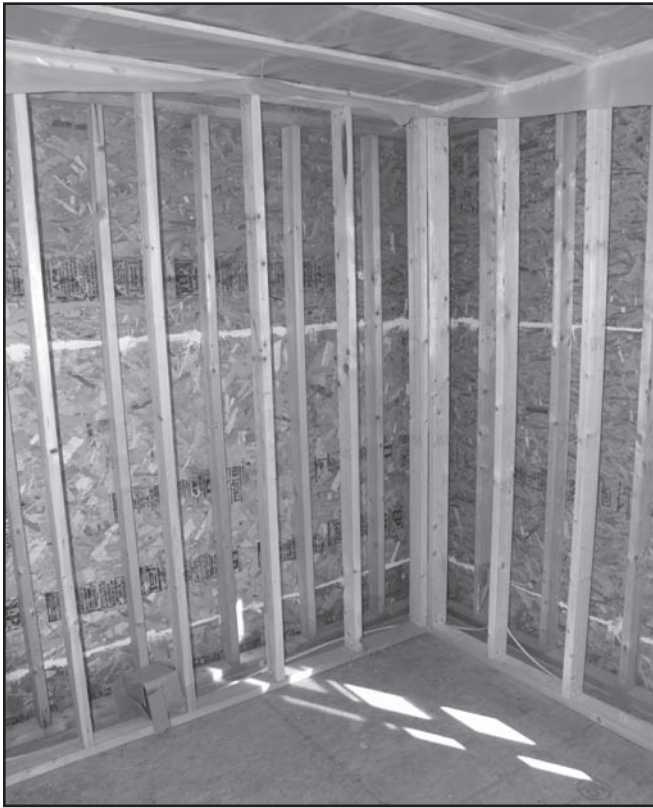
Figure 2. Double walls prior to insulation. Image courtesy Steven Winter Associates.
